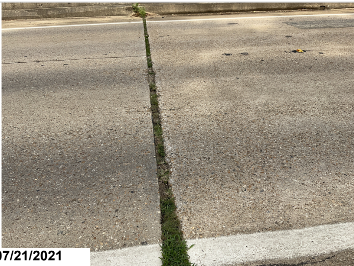
Bent 1 Joint seals have debris impaction.
