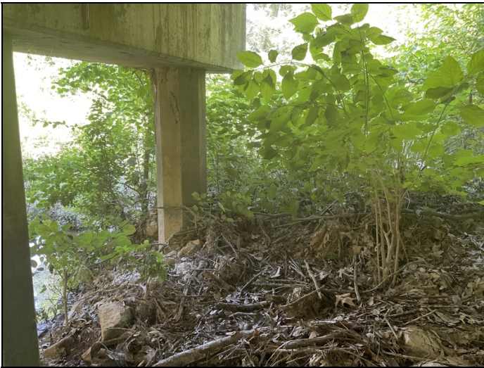
Span 3 left side has trees and vegetation growing under bridge.
