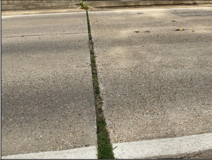
Bent 1 Joint seals have debris impaction.
