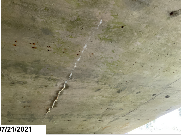
Span1 left side of soffit has cracking with efflorescence.
