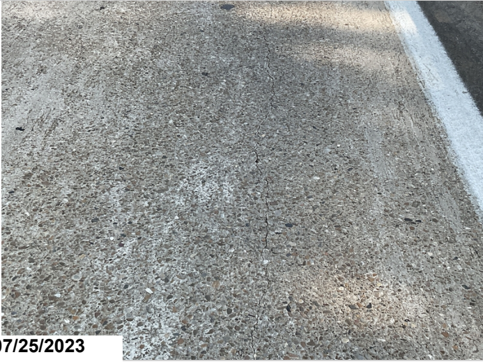
Span 3 deck right lane has large unsealed longitudinal cracks.
