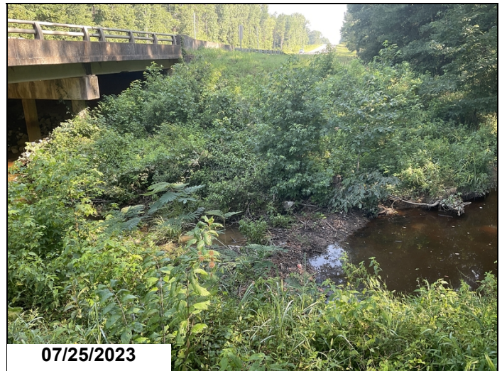
Right side of channel (east) has beaver dam restricting water flow.
